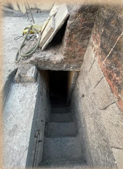
NOT PROPER COVERING TO THR STAIRCASE SO IN RAINEY SEASON RAIN WATER COMES IN SO TO BE PROPERLY COVERED
