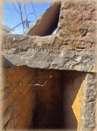
NOT PROPER COVERING TO THR STAIRCASE SO IN RAINEY SEASON RAIN WATER COMES IN SO TO BE PROPERLY COVERED
