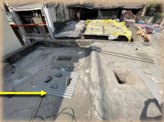
ROOF ABOVE RESIDENCE
