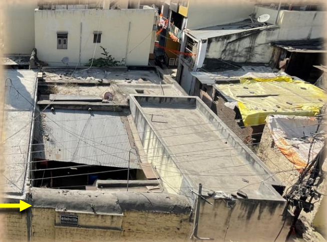
ROOF ABOVE RESIDENCE
